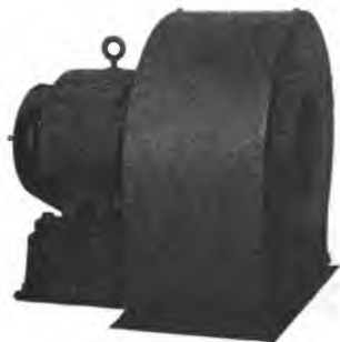
Fig. 4667. 9 1/2-H. P. Motor-Driven Blower for Auto-Transformer. Westinghouse A. C. Electric Locomotive.
